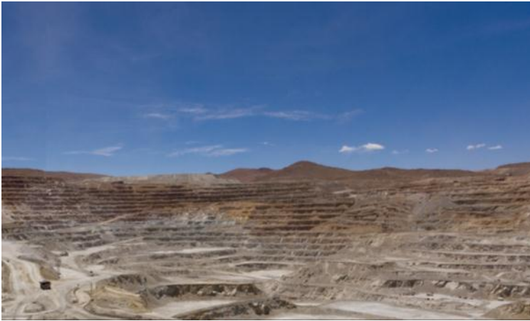
Teck's Quebrada Blanca mine
